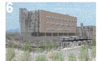
UNM Hospital - Currently under Construction
